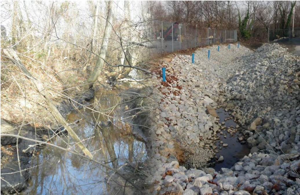
View of the Mecco Drive Ditch Before and After Remediation Activities
